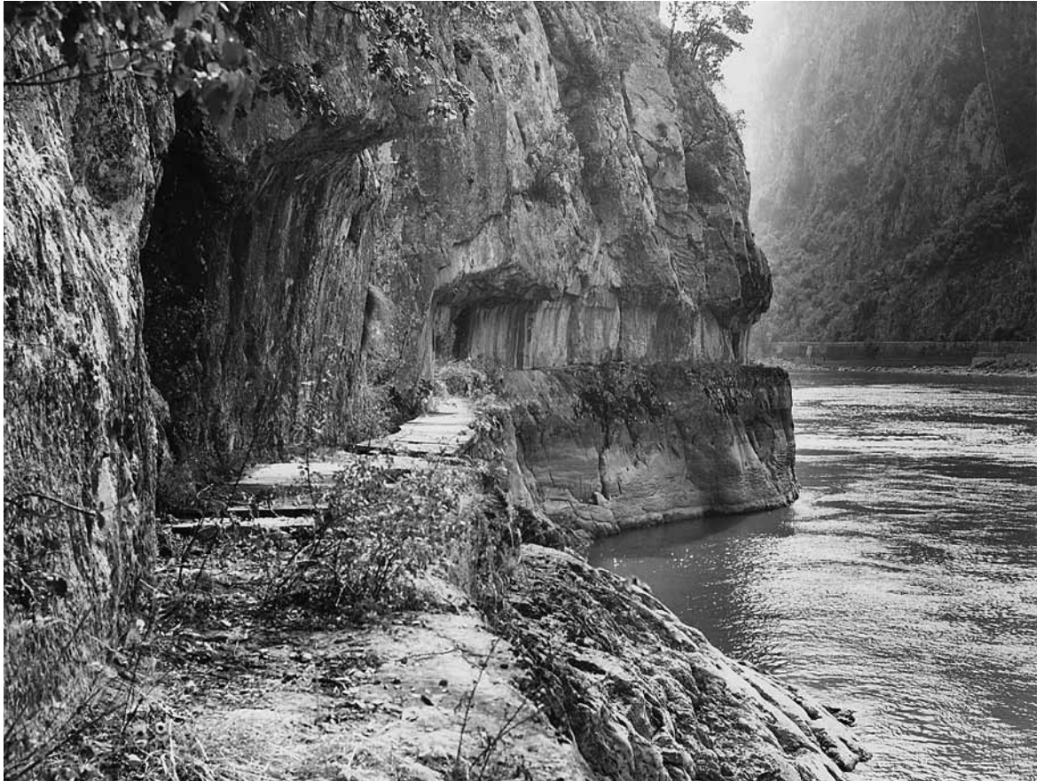
Fig. 3.17 Towpath cut into the rock of the Đerdap (Iron Gate) gorge in the river Danube near Kloadovo, Serbia, before the water level was raised for a hydro-electric power station.
