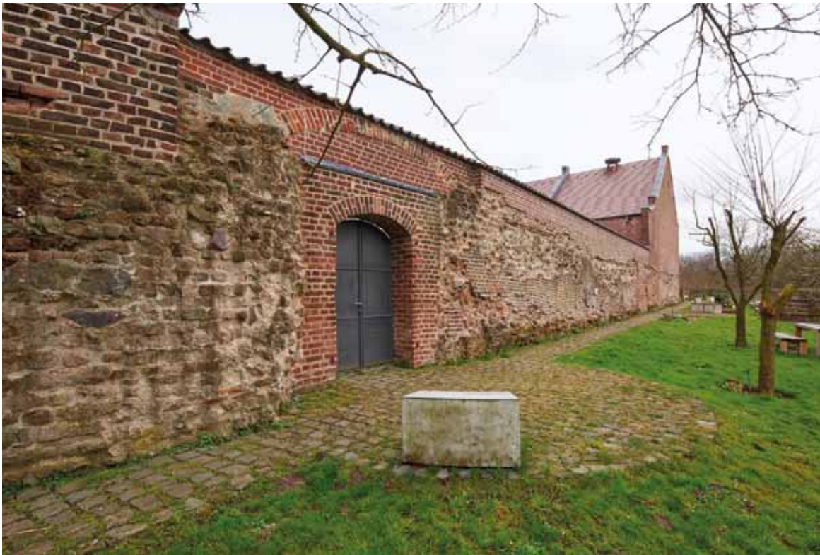
Fig. 4.4 Stretches of original masonry of the Late Roman fortification are still visible in the facade of Haus Bürgel (► 35) today. The fortification's layout is marked out with cobblestones.
