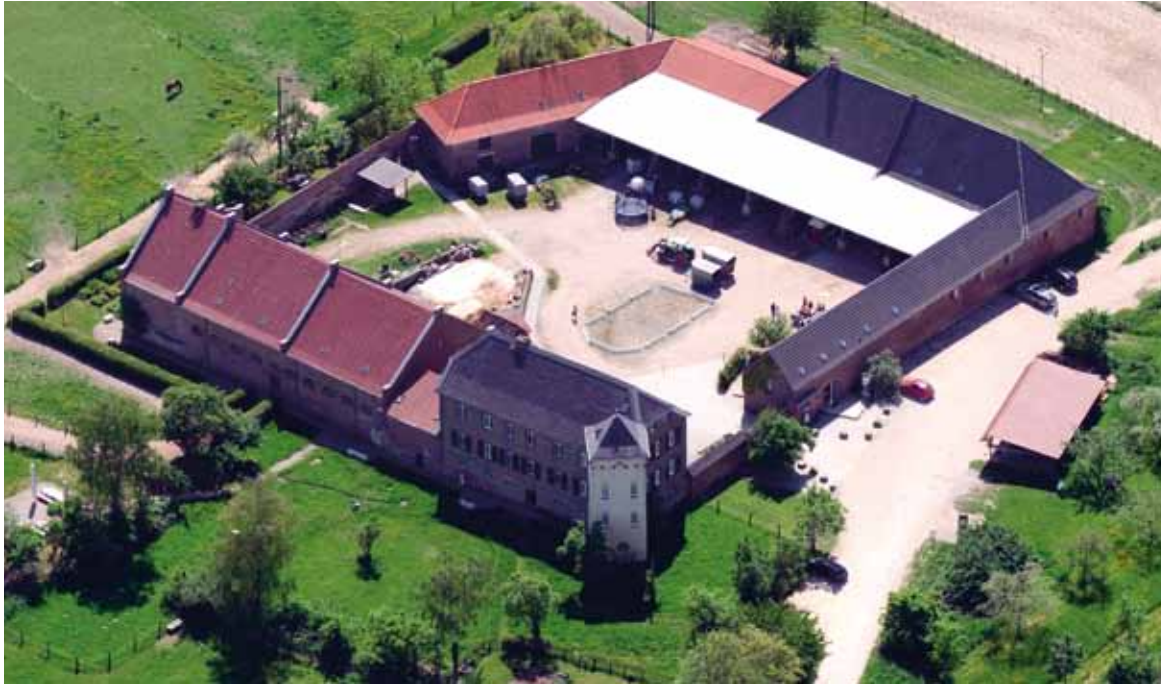
Fig. 2.18 Aerial view of Monheim-Haus Bürgel ▶35. Parts of Late Roman masonry are still visible in the buildings' facade today.
