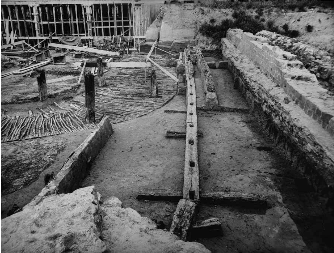
Fig. 2.9 Southwest corner of successive defensive walls of the fort at Valkenburg-Centrum ▶ 1. Left: track of horizontal beams constituting the base of an earthen rampart. Centre: sleeper beams of the fronts of two successive earth-and timber ramparts. Right: collapsed remains of a stone wall.
