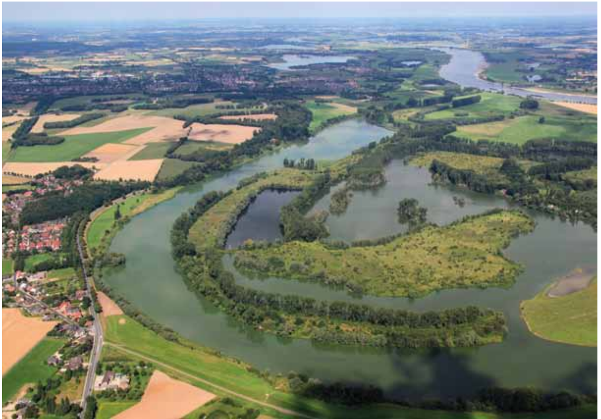
Fig. 4.9 Aerial view of the abandoned gravel extraction on the site of the legionary fortress Vetera II at Xanten.
